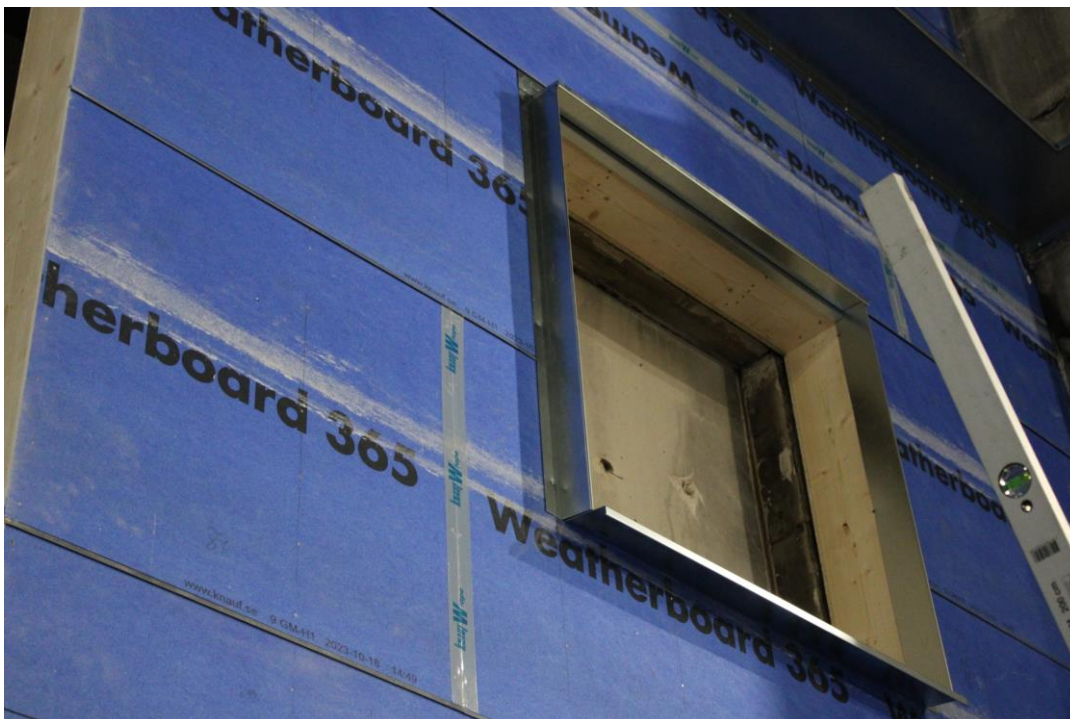
Photo No. 6 Window steel flashing is mounted
