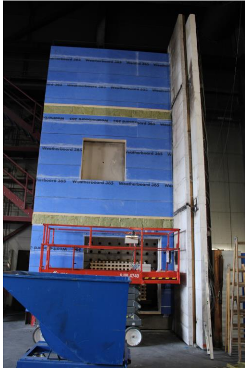
Photo No. 3 Insulation mounted between the prefabricated cassettes
