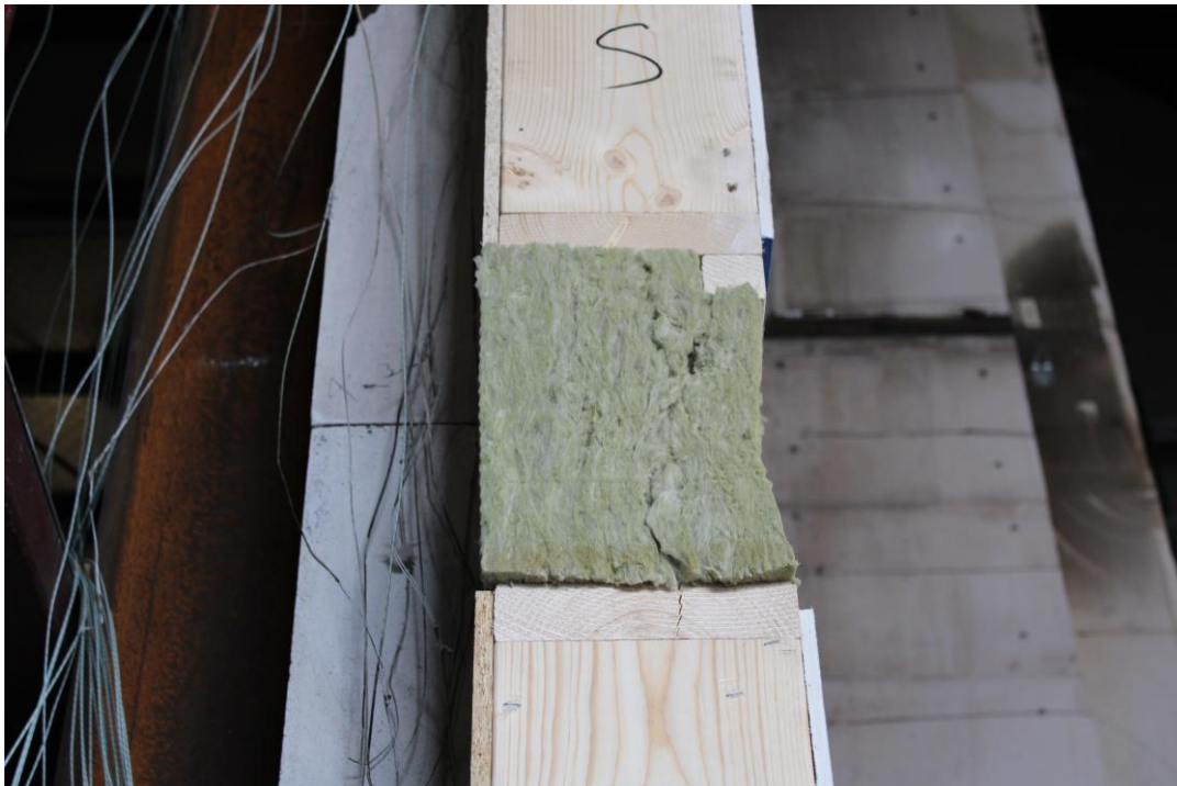
Photo No. 4 Insulation in the gap between two cassettes
