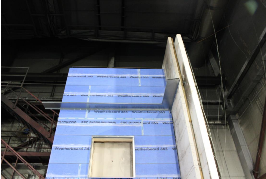
Photo No. 5 Flame deflector is mounted
